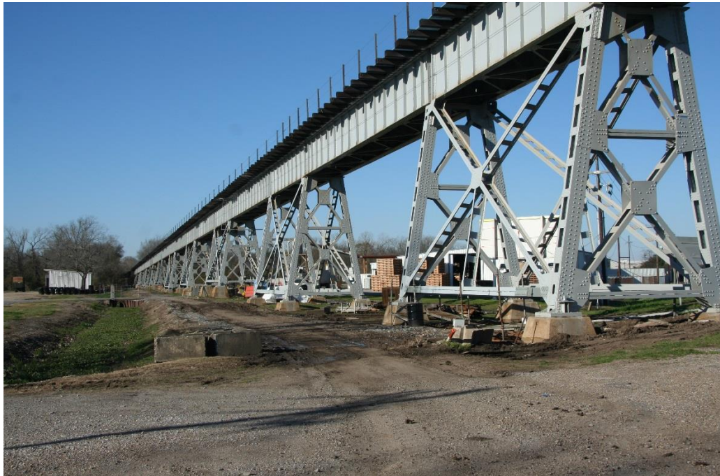
Condition Photo 24: Railroad west approach spans, looking west, repaired and painted.
