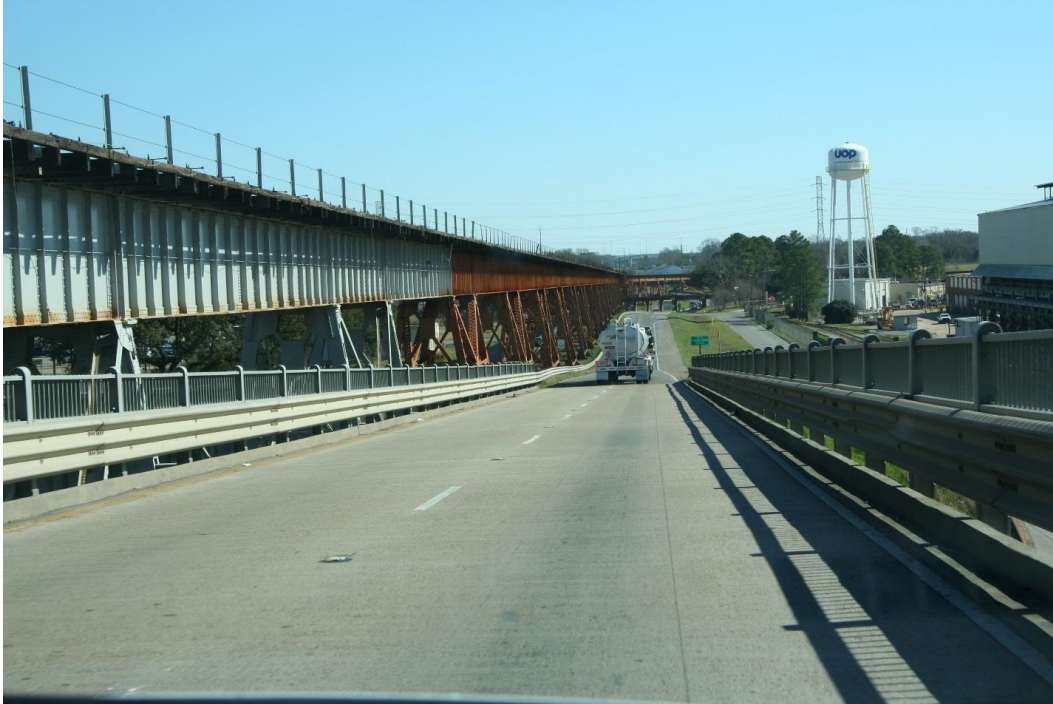
Condition Photo 13: Eastbound roadway off-ramp, looking east. Note progress of cleaning and painting the railroad portion of the bridge (as of February 2016 site visit).
