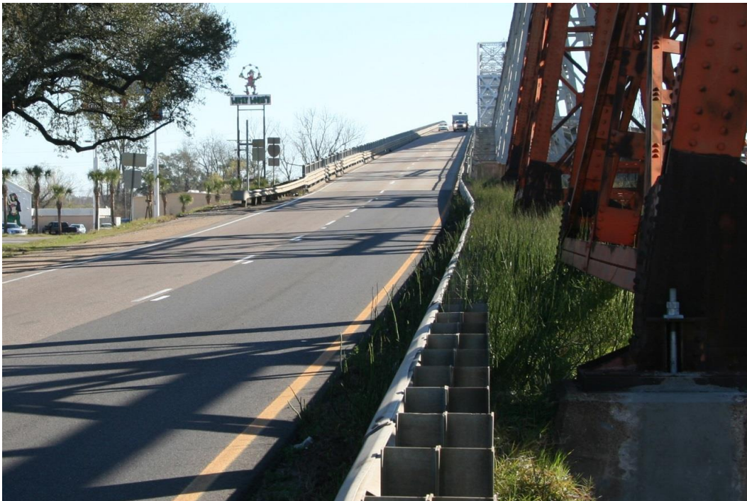
Condition Photo 6: Westbound US 190 exit ramp roadway at west end of bridge, looking east.
