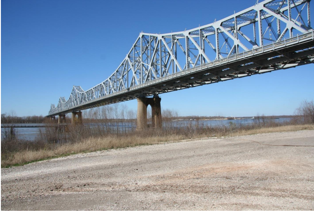
Condition Photo 15: Truss spans, looking northwest.
