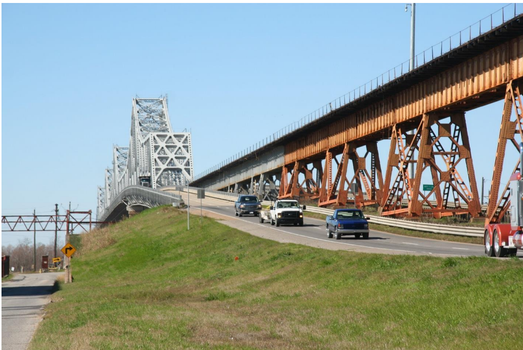
Condition Photo 14: Eastbound roadway off-ramp, looking west along frontage road. Note progress of cleaning and painting railroad portion of bridge (as of February 2016 site visit).
