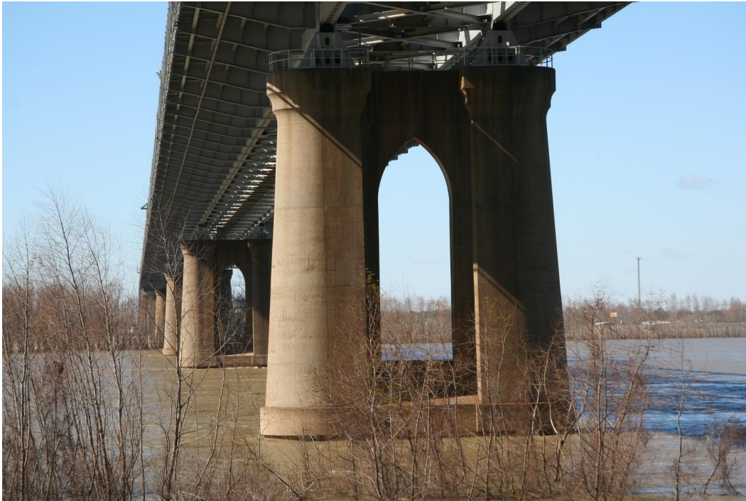
Condition Photo 17: Main river piers 5, 4, 3 and 2 (pier 2 in foreground).
