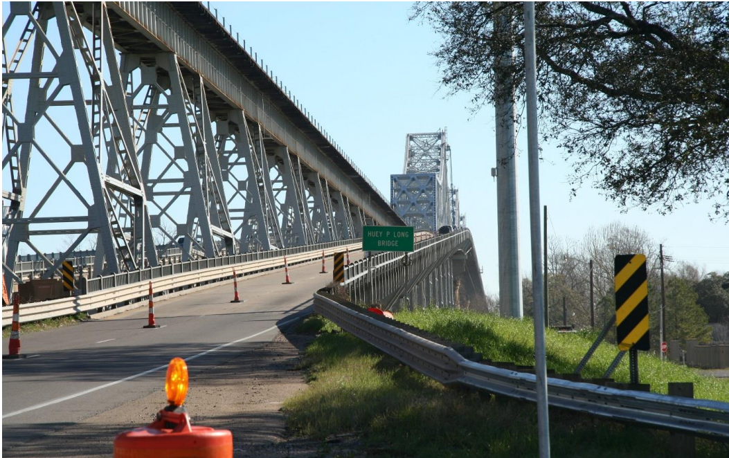
Condition Photo 5: Eastbound US 190 roadway on-ramp approach spans, looking east.
