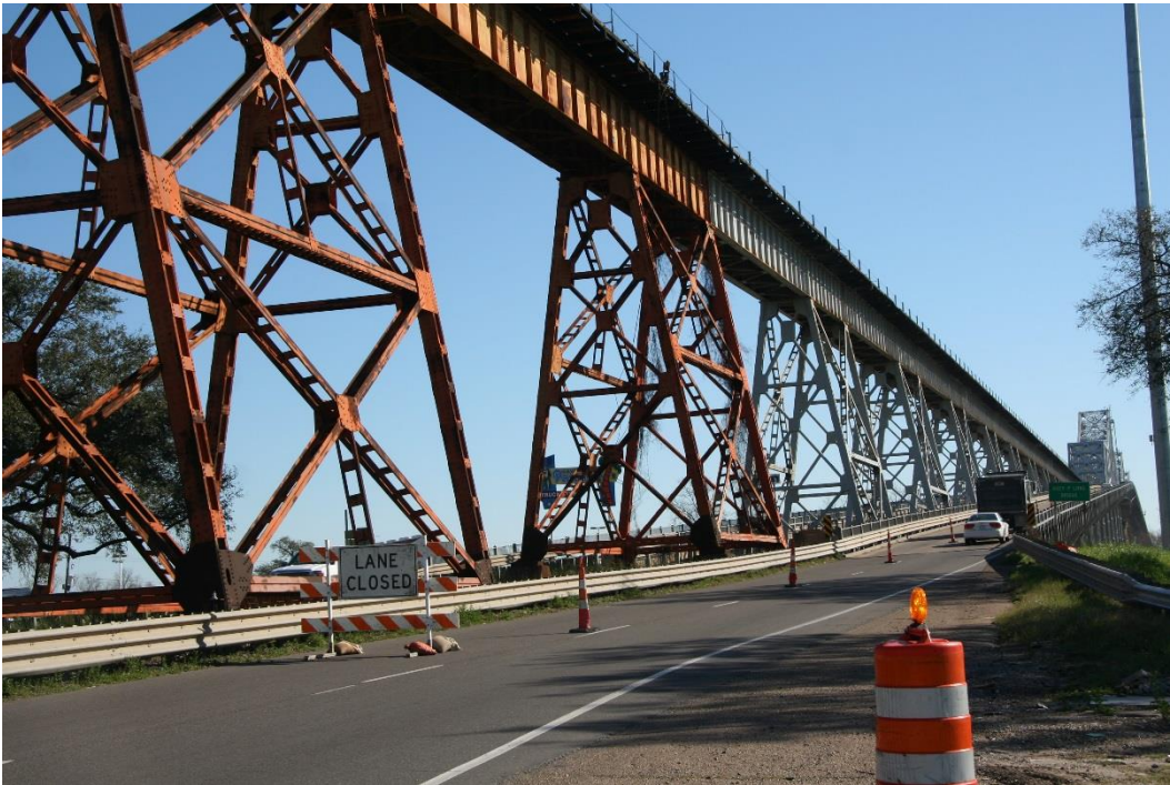
Historic Fabric Photo 1: Railroad approach spans to the west of the main truss spans, including braced steel column substructure.
