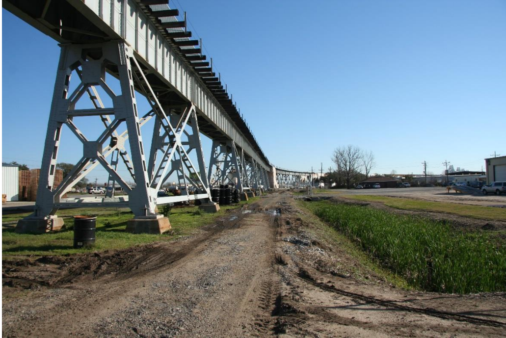
Condition Photo 25: Railroad west approach spans, looking east, repaired and painted.
