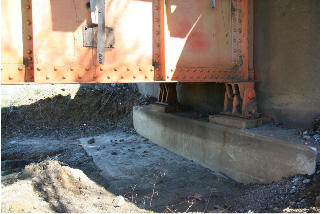
Condition Photo 31: Expansion bearings for railroad girders at east abutment.
