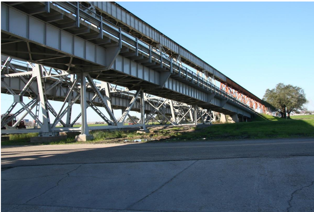
Condition Photo 2: Westbound US 190 exit ramp structure, north side, west end of bridge.
