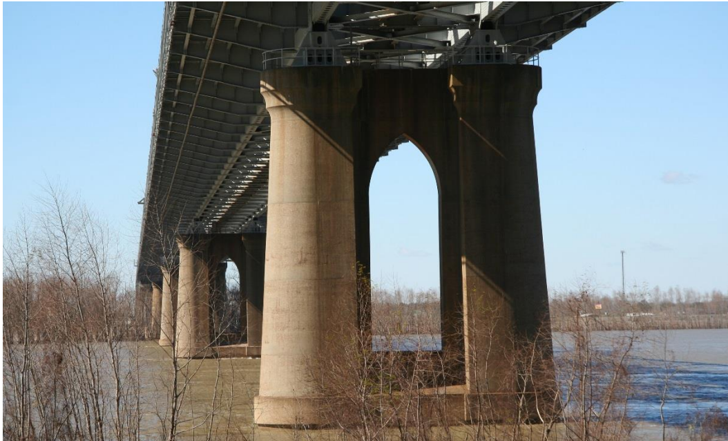
Character-defining Feature Photo 3: Caisson-constructed piers.
