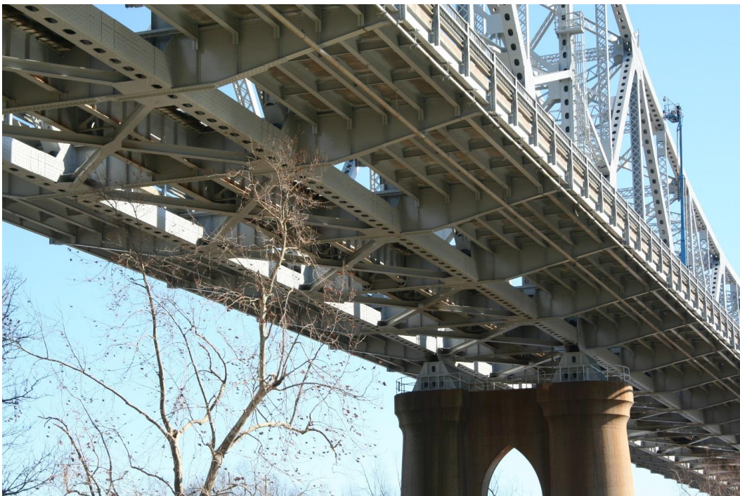
Condition Photo 10: Truss span at pier 2, looking east.
