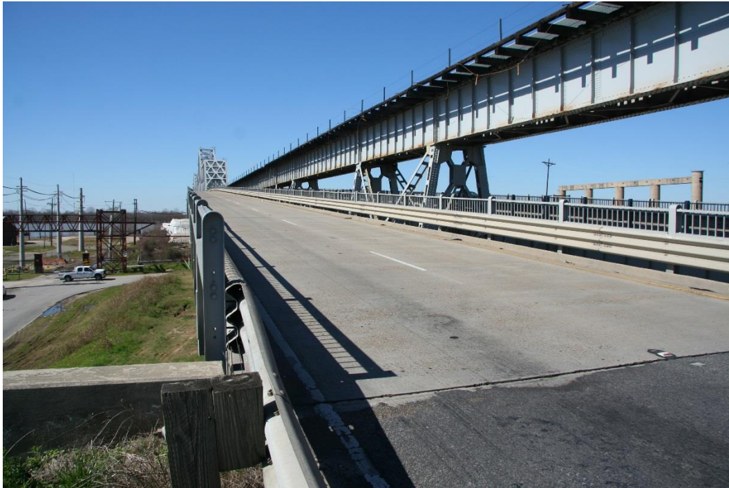
Historic Fabric Photo 3: Original bridge railings along the easterly approach spans.
