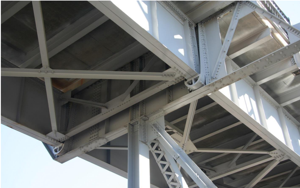
Condition Photo 3: Steel girder span expansion bearings at braced steel bent.
