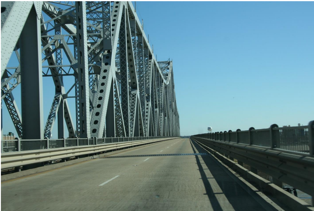
Condition Photo 12: Eastbound roadway across truss span, looking east.
