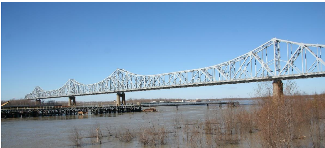
Character-defining feature Photo 1: Design and construction of a continuous and cantilevered Warren through truss.
