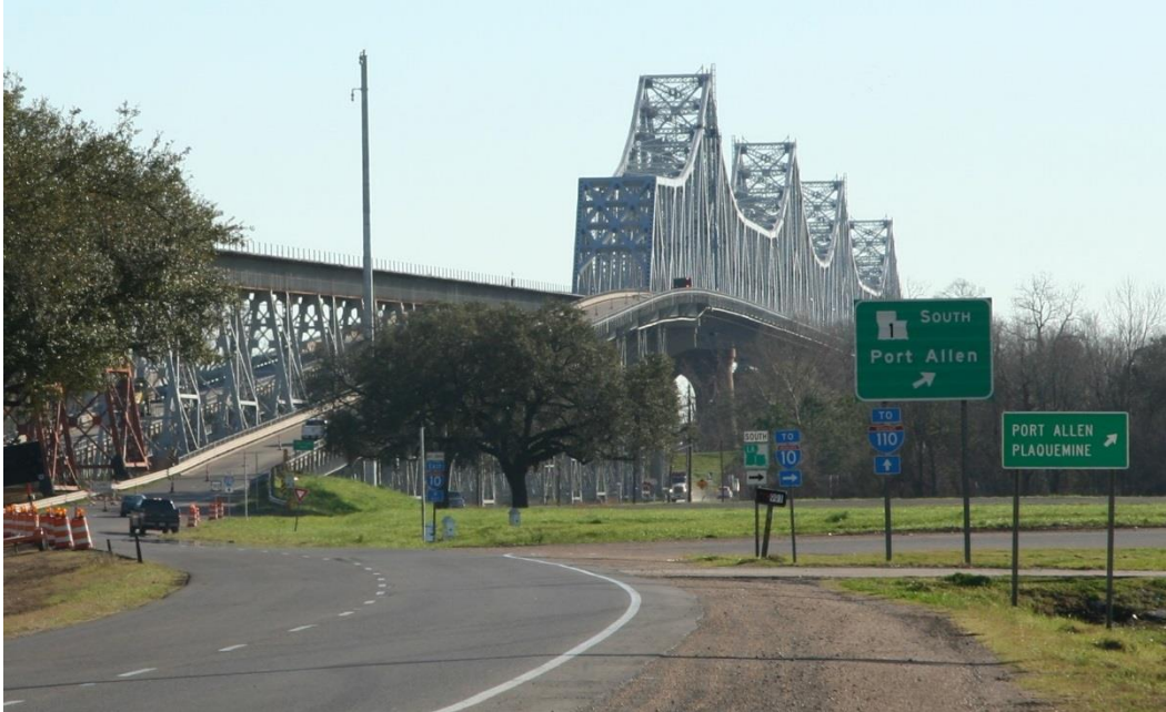
Condition Photo 1: Overview of bridge looking east, with highway signage and entrance ramp to go east on US 190.
